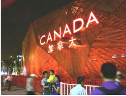
The Canada Pavilion, Exterior
